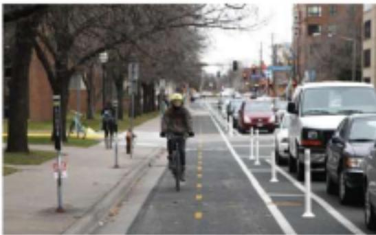
*Delineator-protected bikeways use plastic delineator posts or “bollards” and a painted buffer space between the bikeway and the travel or parking lane to provide physical separation from motorized traffic. This photo shows a delineator-protected bikeway along Oak Street SE in Minneapolis.*
